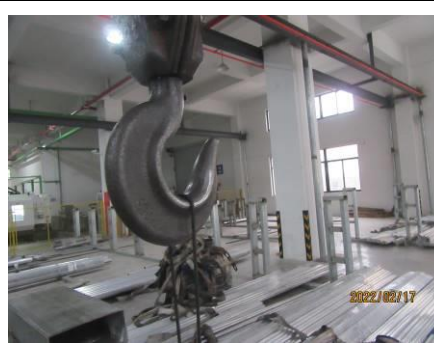
NC photo 2: No safe lock was installed for the hooks of one crane.
