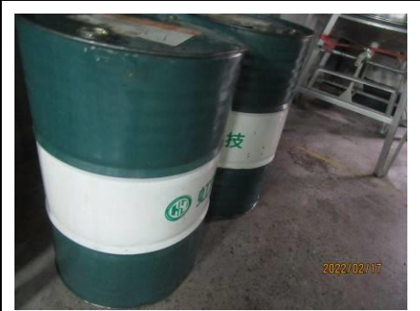
NC photo 3: Insufficient anti-leakage facility.
